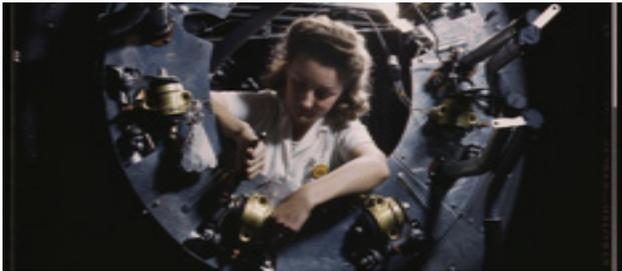
Part of the cowling for one of the motors for a B-25 bomber is assembled in the engine department of North American [Aviation, Inc.]'s Inglewood, Calif., plant. 1942
